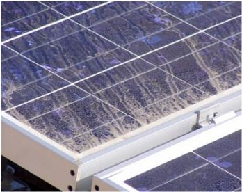
Fig. 2 Dust fall on solar panels.
